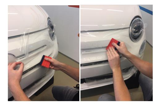
• For curved areas, it is necessary to firmly pull and stretch the film in order to conform the film around the surfaces. It is recommended to stretch the material without applying any heat, making use of the intrinsic flexibility of the Paint Protection Film. Make sure not to overstretch the material to the point of creating white lines into the face film.
