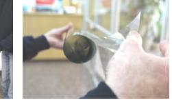
Step 4 Spray the exposed adhesive layer with plenty of wetting solution, and on the clean glass.
